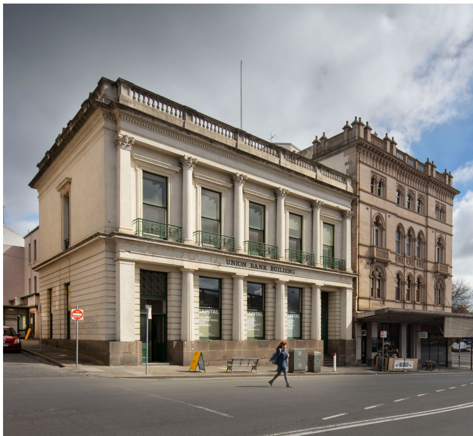
Future home of the National Centre for Photography Photo: John Gollings, 2019
